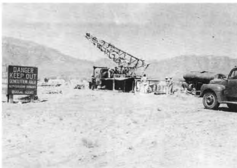
FIGURE 2.- Rotary drilling rig being assembled at site of well R-28.
