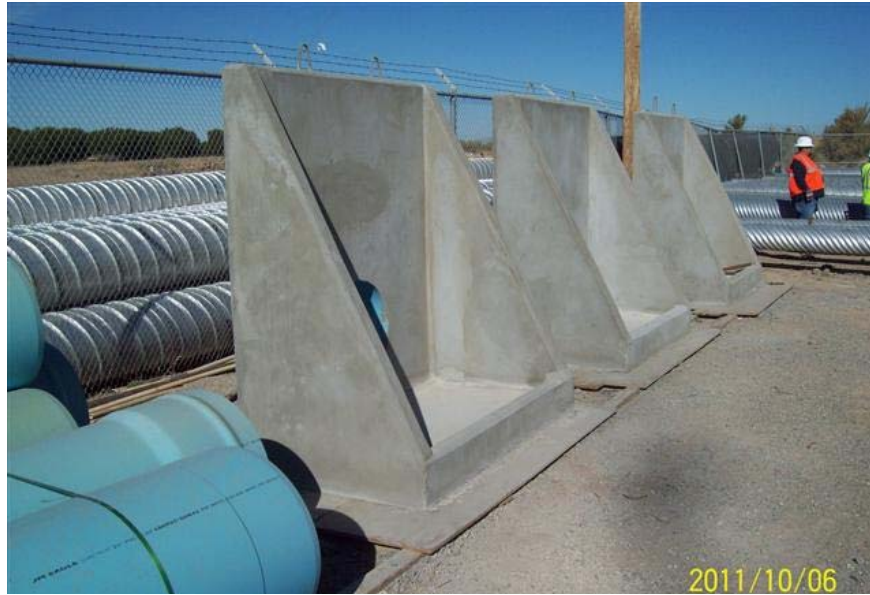
Figure 2. Construction of 24” Headwalls
