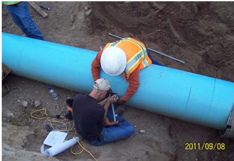
Figure 4. Installation of ultrasonic transducer at Bills Farm
