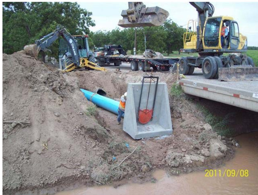
Figure 3. Installation of 24” Headwall at 26.98R Franklin Canal
