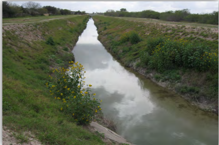
Photo 20. Outfall SW3 discharge area. View to the south.
