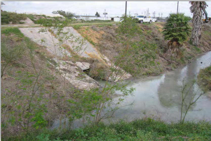
Photo 3. Outfall SE1. View to the northwest.
