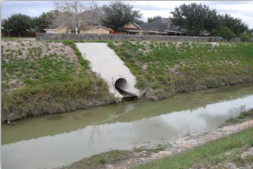
Photo 29. Outfall SW8. View to the northeast.
