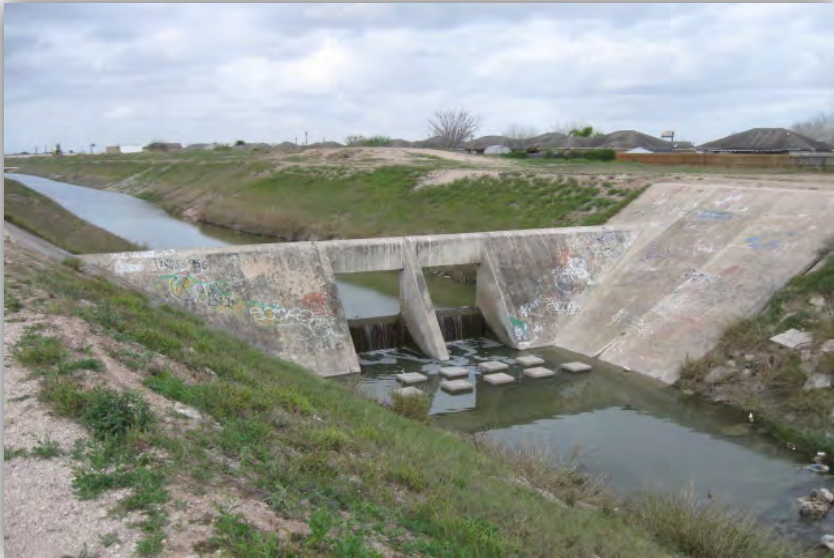
Photo 1. Outfall SE2. View to the west.
