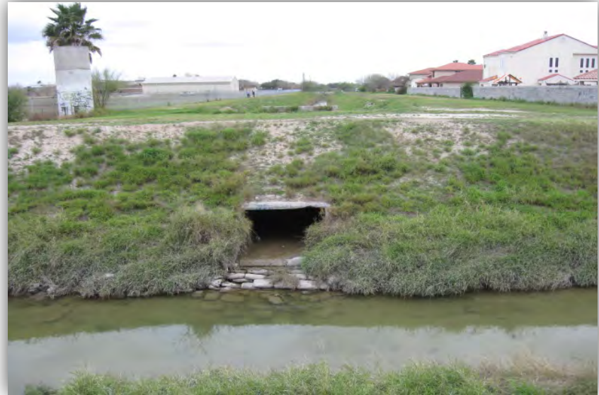
Photo 22. Outfall SW4. View to the east.
