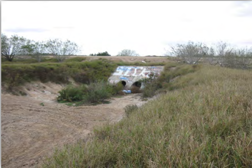
Photo 9. Outfall NW1. View to the east.
