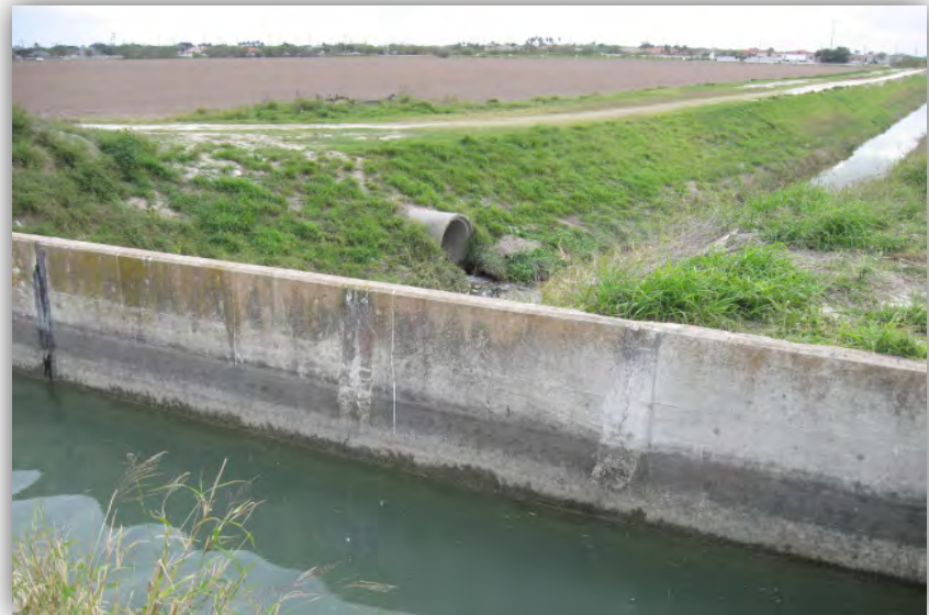
Photo 24. Outfall SW5. View to the southeast.
