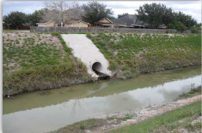
Photo 28. Outfall SW7. View to the northwest.
