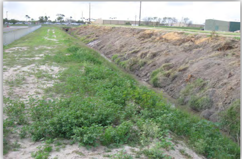
Photo 4. Outfall SE1 discharge area. View to the south.
