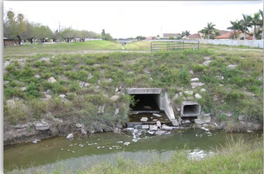
Photo 26. Outfall SW6. View to the south.
