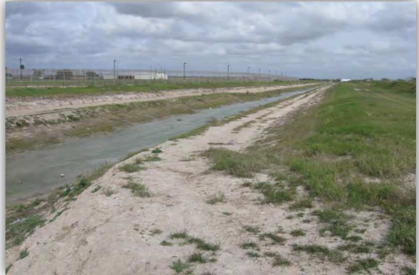
Photo 6. Outfall NE1. View to the north.
