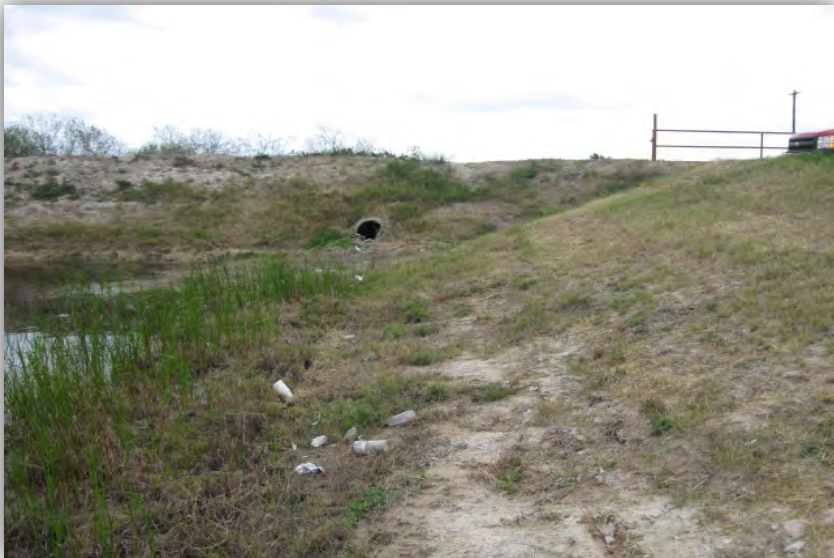
Photo 7. Outfall NW2. View to the east.
