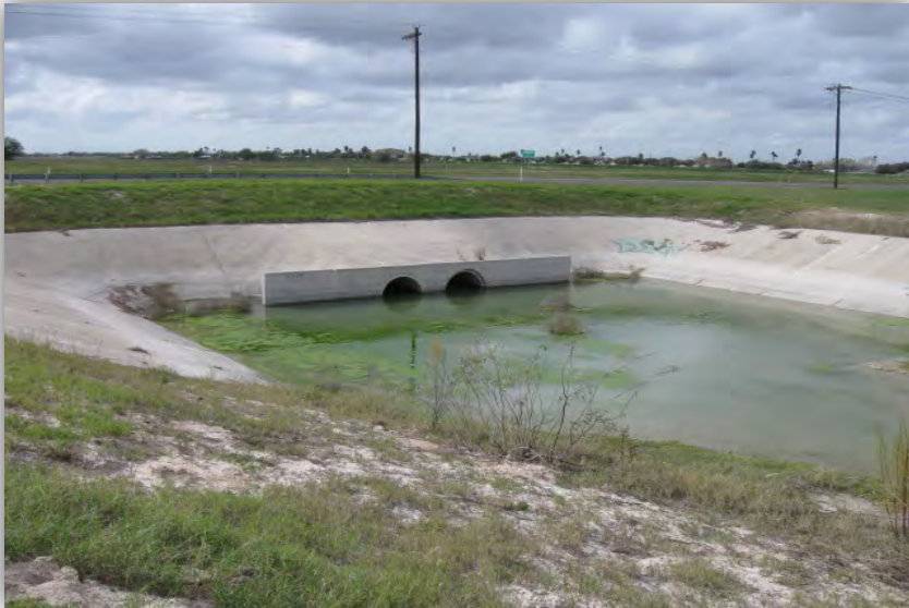
Photo 5. Outfall NE1. View to the southwest.
