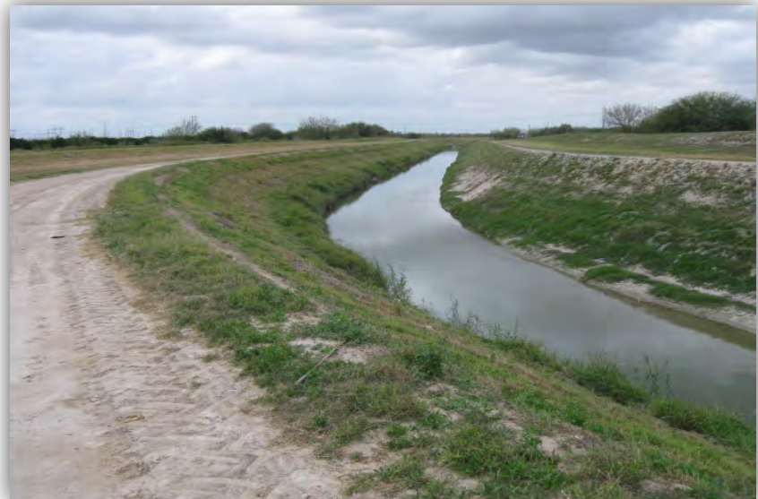
Photo 12. Outfall NW3. View to the west.
