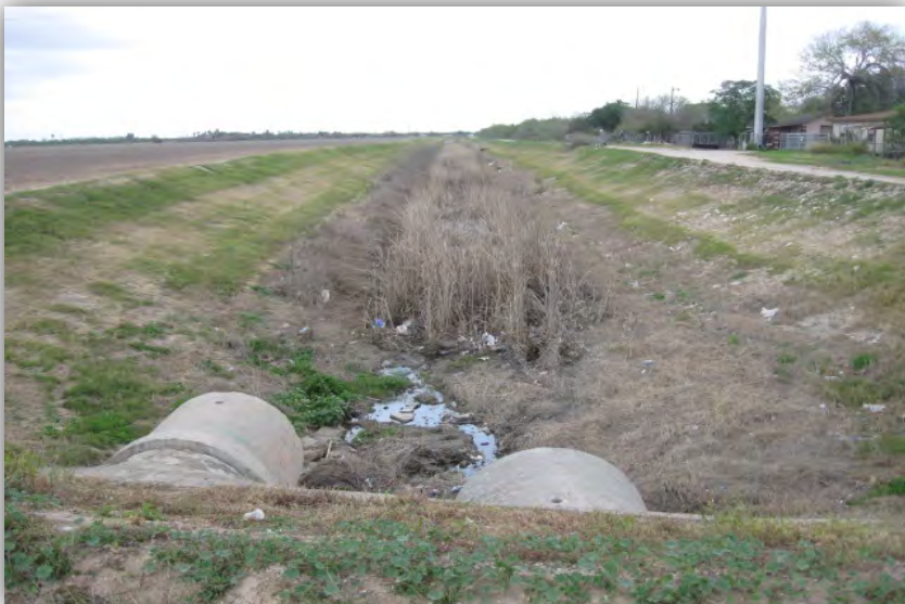
Photo 11. Outfall NW4. View to the north.
