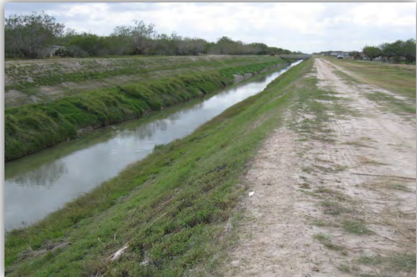
Photo 14. Outfall NW5 discharge area. View to the south.
