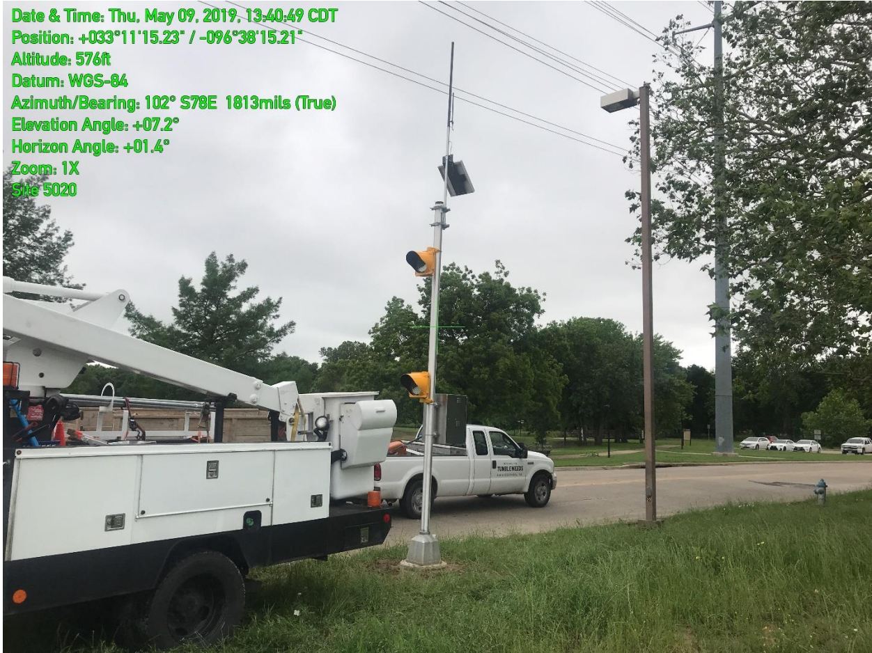
Figure 5. Installation of Remote 2, Park View East
