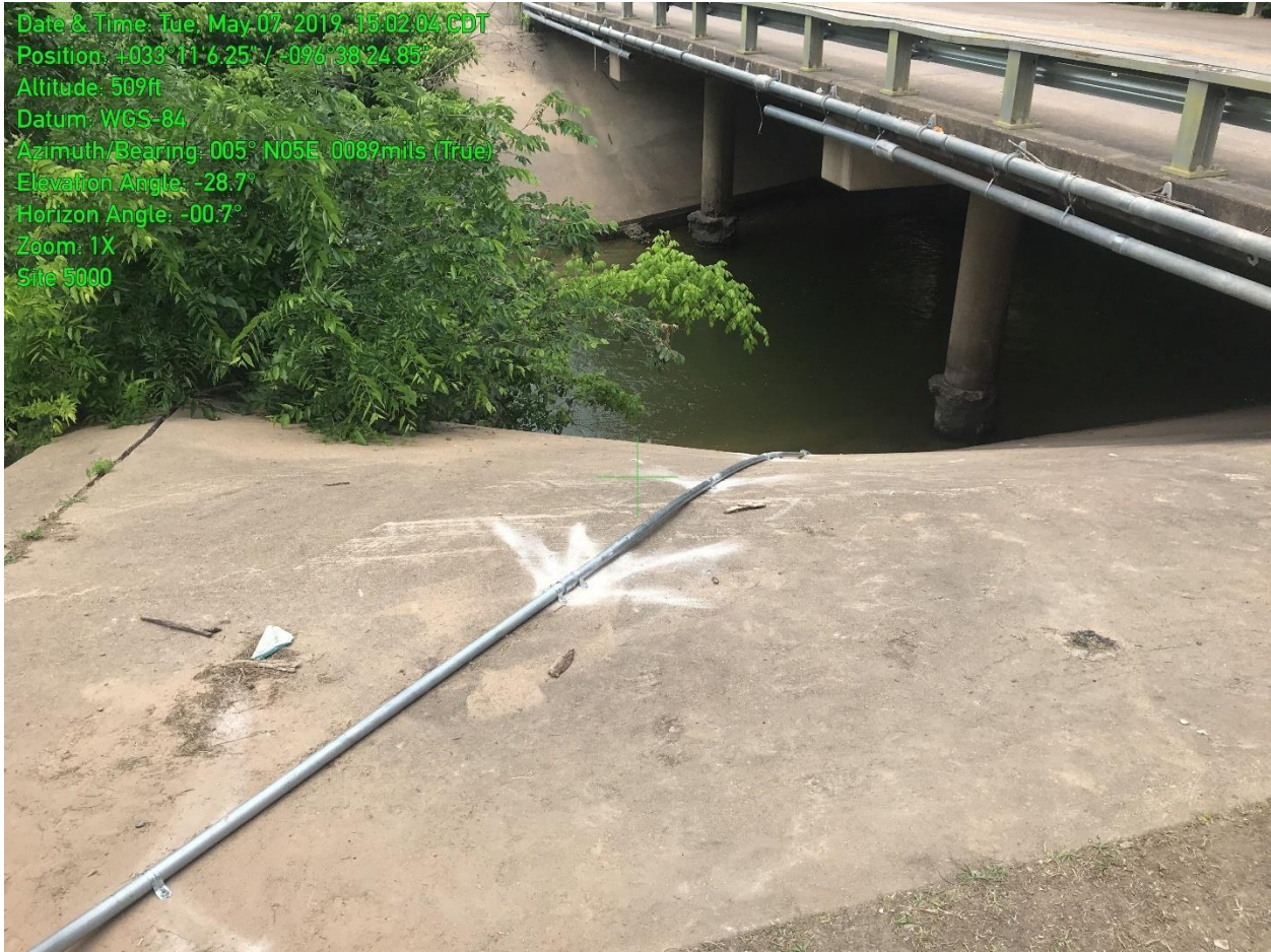
Figure 7. Installation of the Pressure Transducer, Wilson Creek
