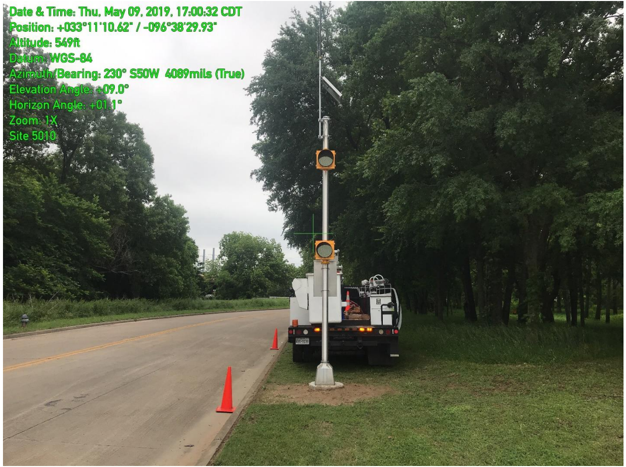
Figure 4. Installation of Remote 1, Park View West
