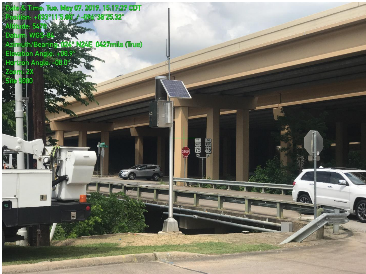
Figure 6. Installation of Master Gauging Station, U.S. 75 and Wilson Creek Bridge
