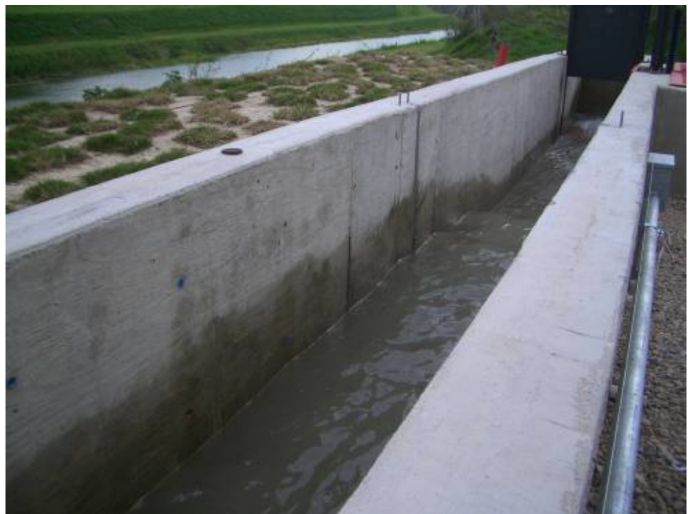
Water over Broad Crested Ramp at a rate of 6.5 cfs
