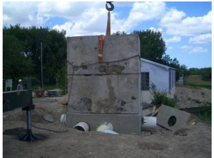
Setting the Concrete Boxes
