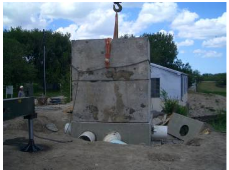
Setting the Concrete Boxes
