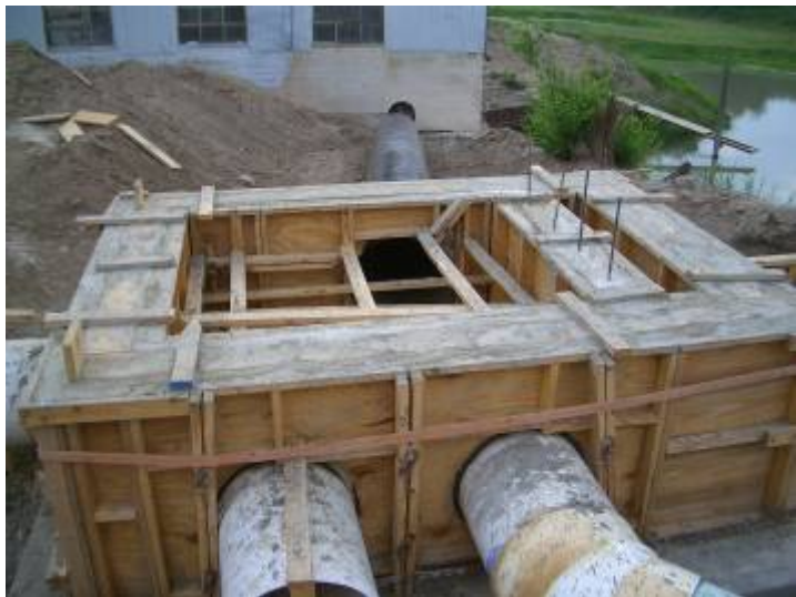
Diversion Box Foundation
