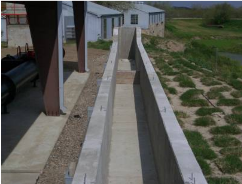
Flume inlet with Sharp Crested Weir
