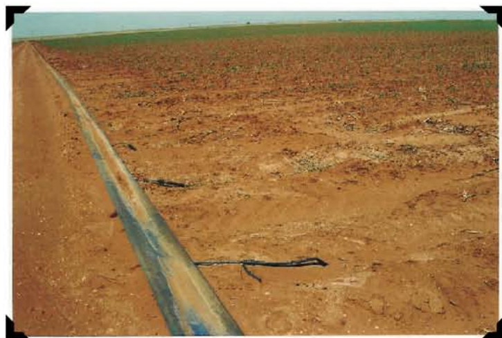
Lay flat and drip line connected.
