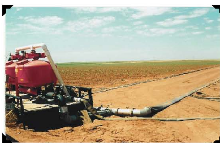
The "lay flat" lines are connected to the filter system. Individual rows of underground drip line are then connected to the "lay flat."
