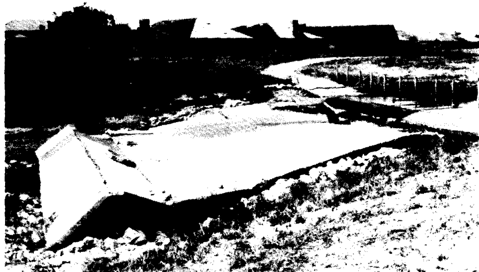
Sikes Lake Spillway and Concrete Apron
