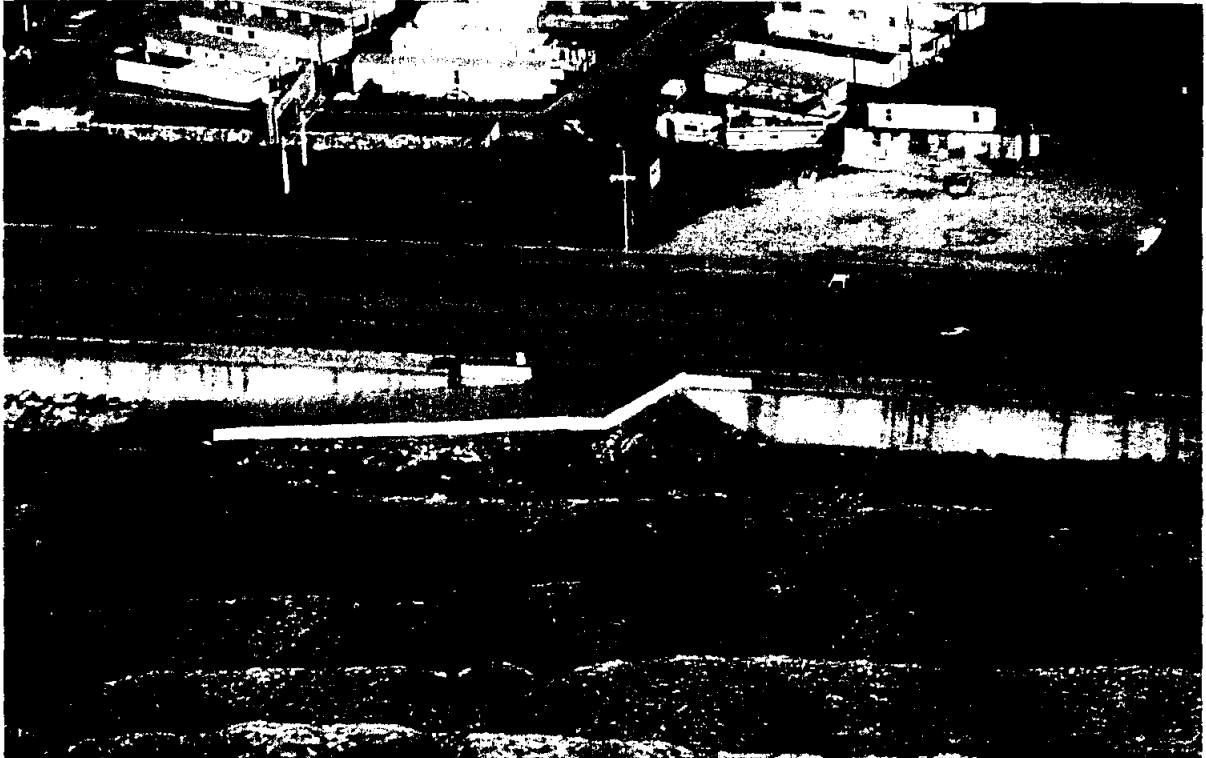
GALVESTON - 59TH STREET: SEAWALL DOWN RAMP TO NO BEACH
