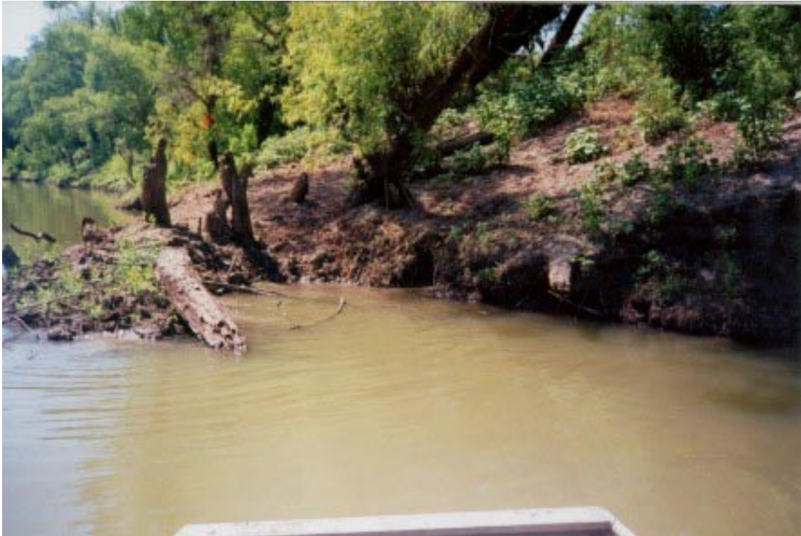
Figure 6. Site 2. A-19 on left, B-18 on right. Upstream view.
