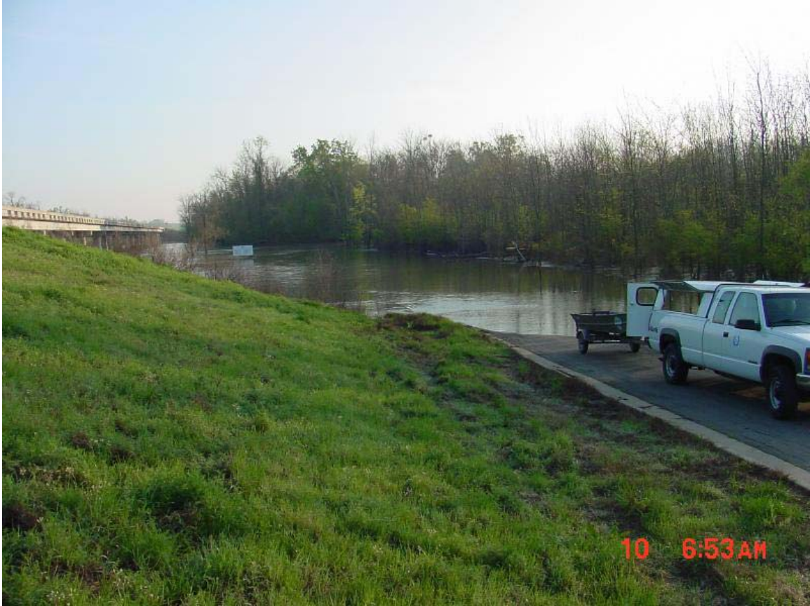
Figure 6.8– Photo of inundation in an unchannelized section at high flow at upstream boundary of Site 2, April 10, 2002 (297.3 cms, 10,500 cfs at Talco).
