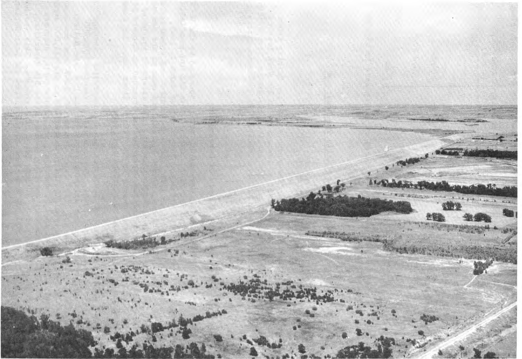
Lewisville Dam and Garza-Little Elm Reservoir. Furnished by U. S. Army Corps of Engineers, Fort Worth District.
