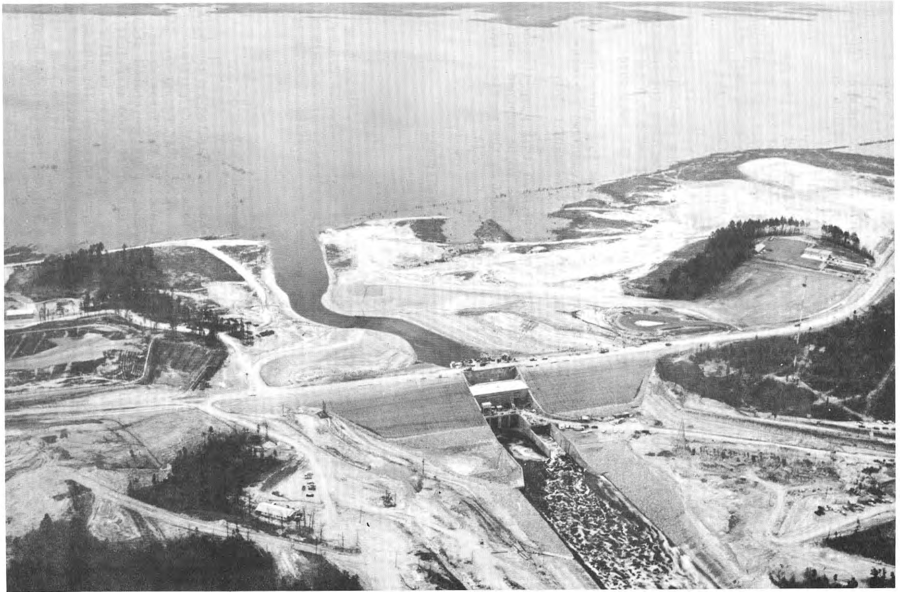
Sam Rayburn Dam and Sam Rayburn Reservoir. Furnished by U. S. Army Corps of Engineers, Fort Worth District.
