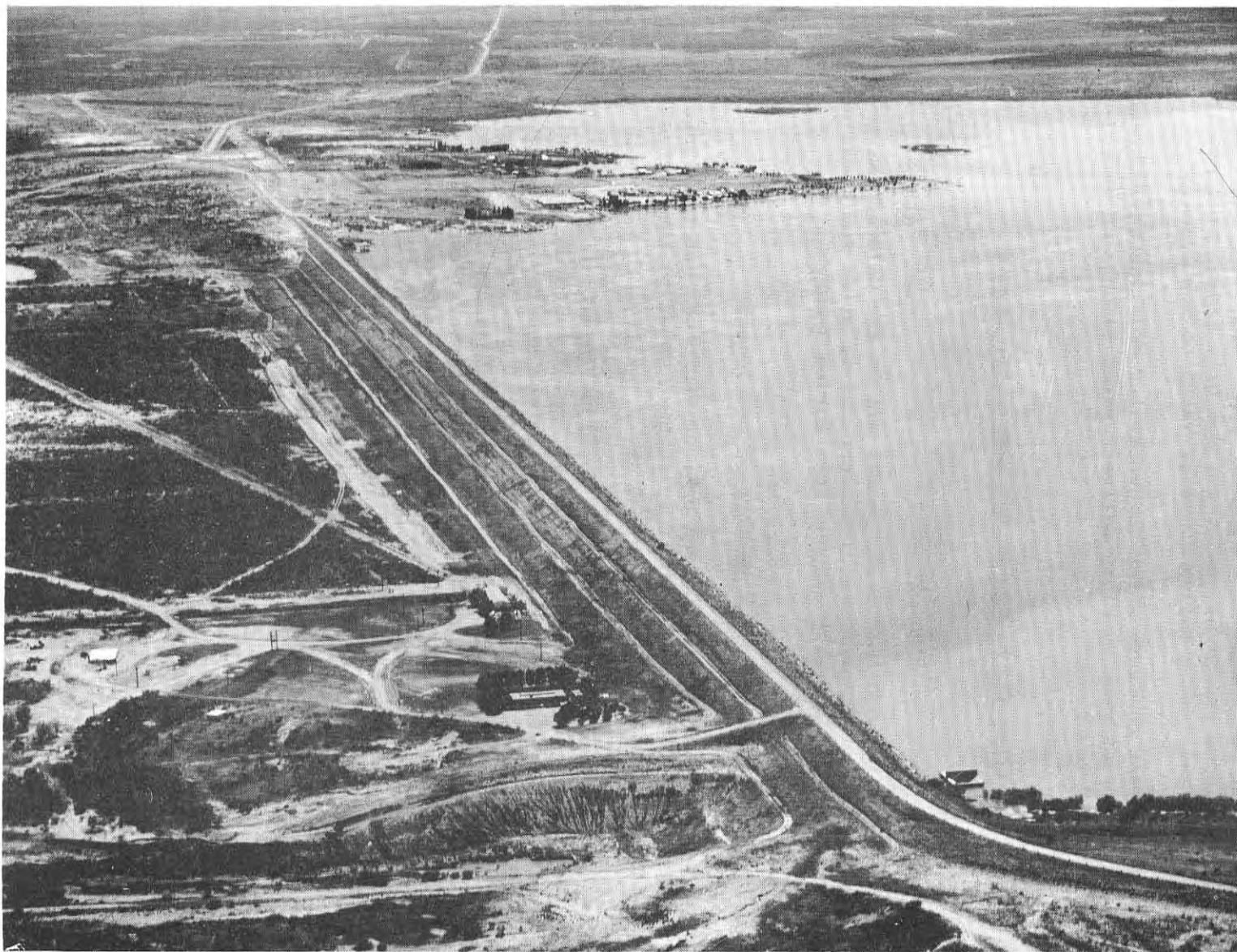
Colorado River Dam and Lake J. B. Thomas. Furnished by Colorado River Municipal Water District.
