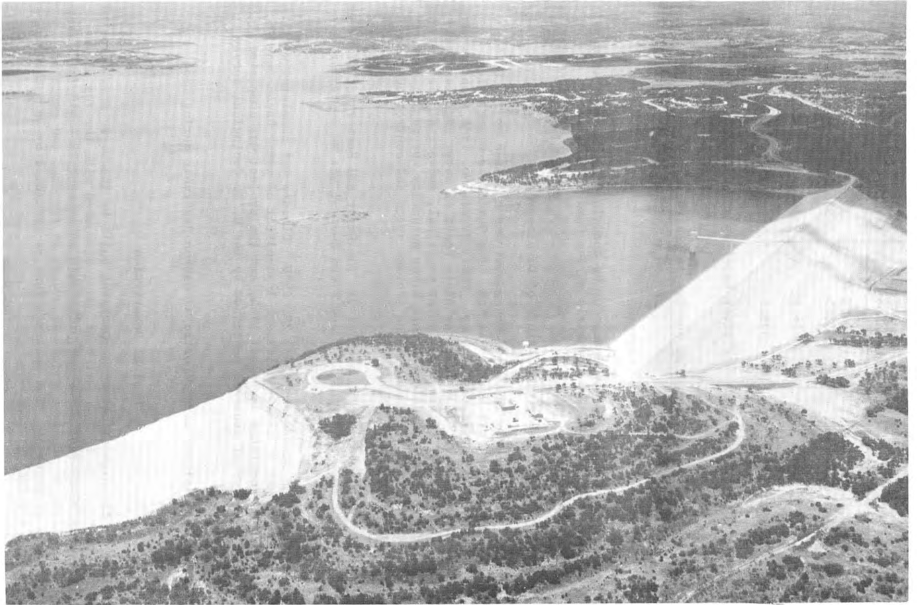
Canyon Dam and Canyon Reservoir. Furnished by U. S. Army Corps of Engineers. Fort Worth District.
