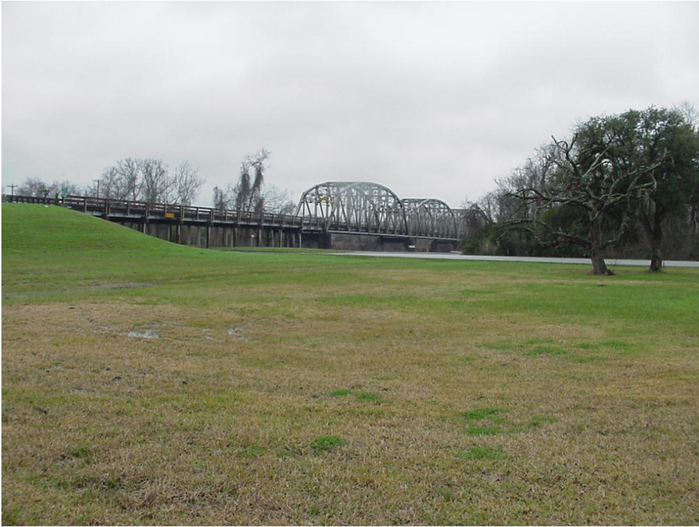
Figure 8 – Photo illustrating elevated highway across Brazos flood plain.
