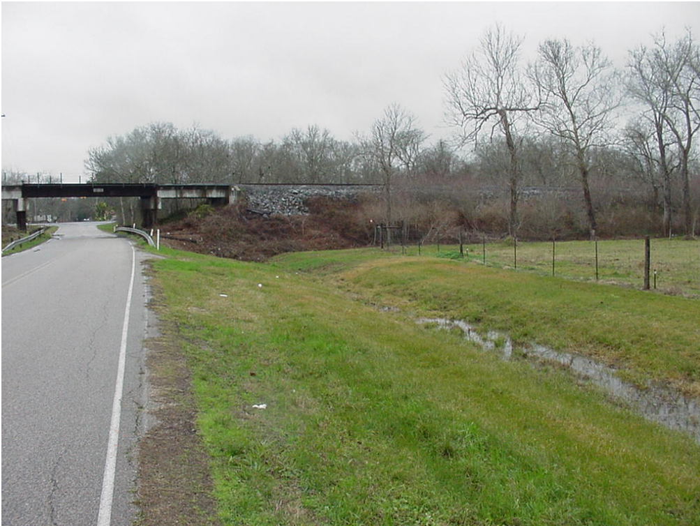
Figure 9– Photo illustrating elevated railway across Brazos flood plain (adjacent to Brazos River).
