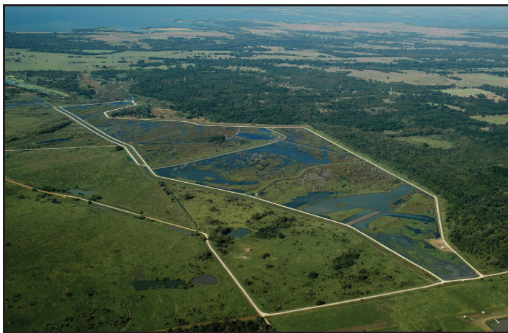
TRWD’s George W. Shannon Wetlands Water Recycling Facility
